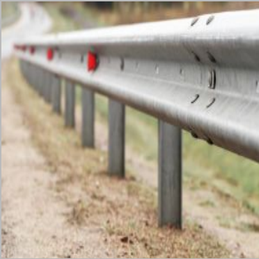
Road Guard Rail
