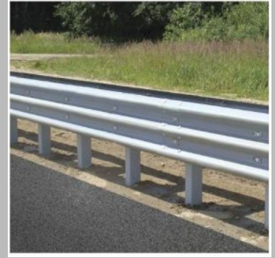
Road Guard Rails
