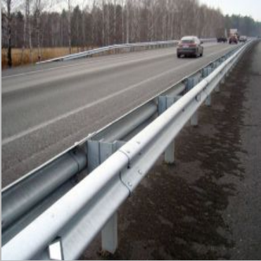
W Beam Crash Barrier Maintenance Services
