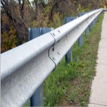
Road Guard Rails Maintenance Service
