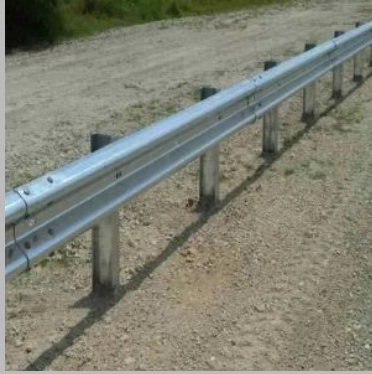
W Beam Crash Barrier
