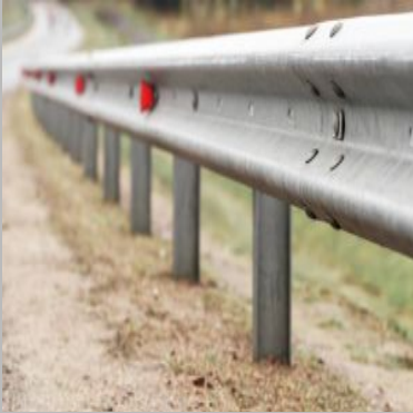
Road Guard Rail
