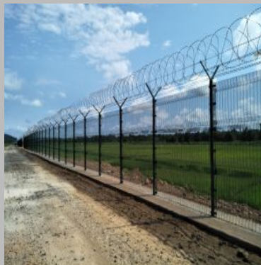
Anti Climb Fence
