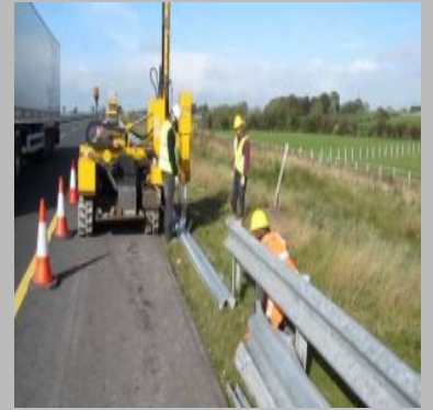
Crash Barrier Installation Service
