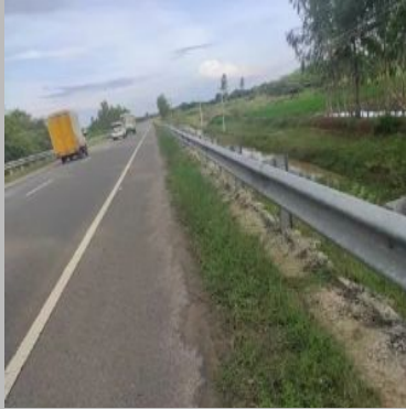
Road Guard Rails Installation Service
