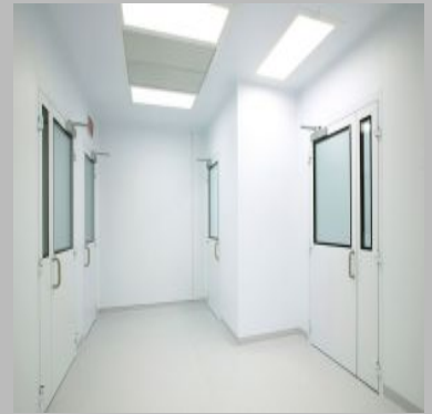
Clean Room Panels
