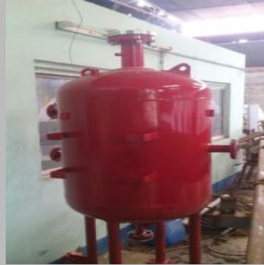
Foam module for rim seal fire protection system
