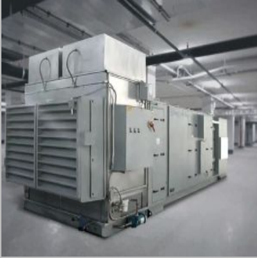
Indirect Evaporator Air Cooling
