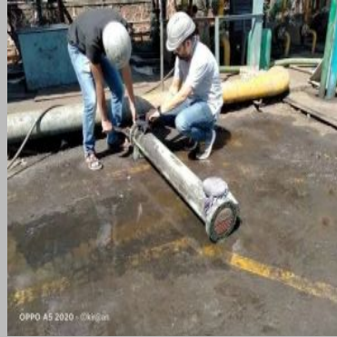
Shell & Tube Heat Exchanger Repairing Services
