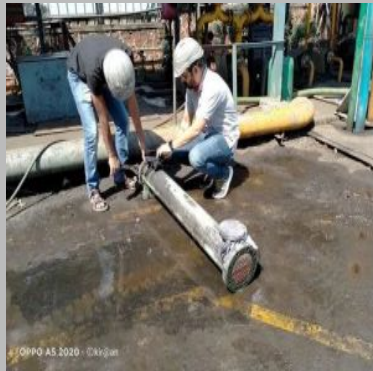
Refurbishment Heat Exchanger
