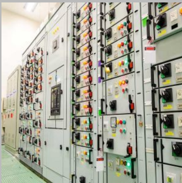
Electrical Panel Installation Services
