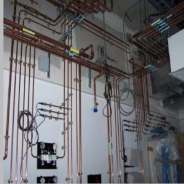
Medical Gas Pipeline Installation Services
