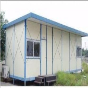
Prefabricated Guest House
