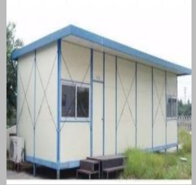
Prefabricated Guest House
