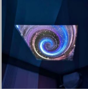
University Stretch Ceiling
