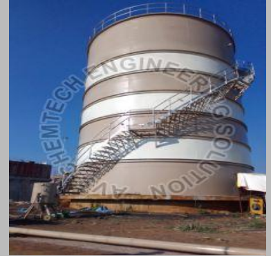
High Capacity Storage Tank
