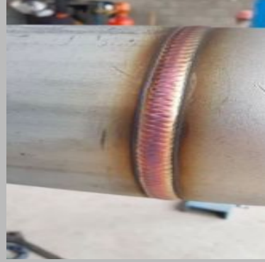
pipe line fabrication
