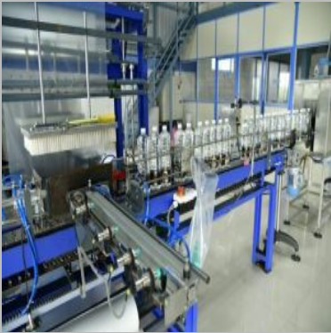
mineral water bottling plant
