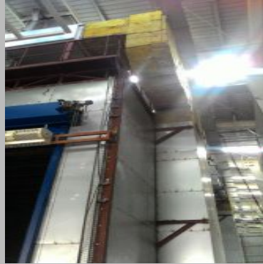
Cladding Ducting Work
