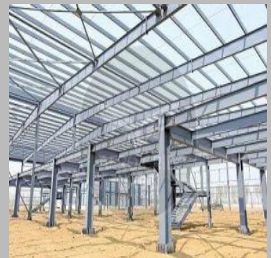
Structural Steel Estimation Services
